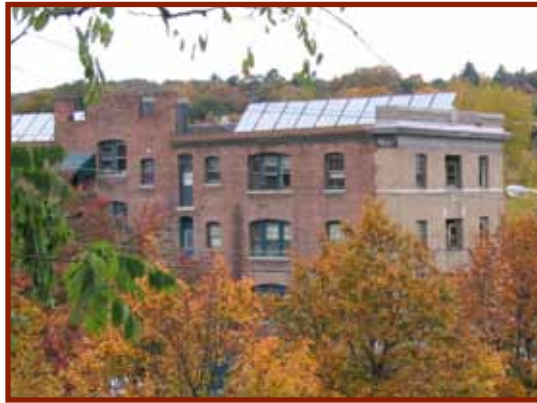
At the Abbott Block in Brattleboro, Vermont, solar panels are expected to save 50 percent annually on domestic hot water. The panels preheat the water supply for 17 apartments, including 2 units in an adjacent building. Other improvements included new energy-efficient windows with low-E glass, 9 inches of hard insulation added to the roof, new ENERGY STAR® appliances, low-flow plumbing fixtures and laundry equipment, and new lighting fixtures and bulbs. Overall, energy retrofit work is expected to save 25–30 percent in operating costs. Photo provided by Windham Housing Trust.
