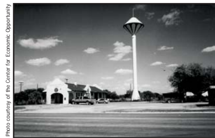
MHWSC built this elevated water storage tank in Colonia Progreso, Texas.
